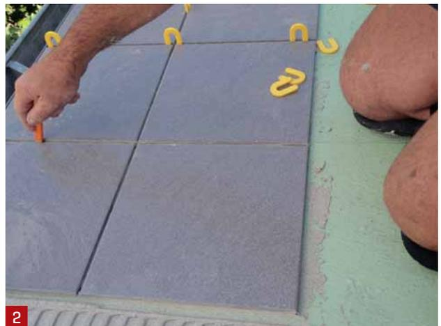
**IMAGE 1:** Lippage between floor tiles. **IMAGE 2:** Cleaning adhesive from movement joints.
